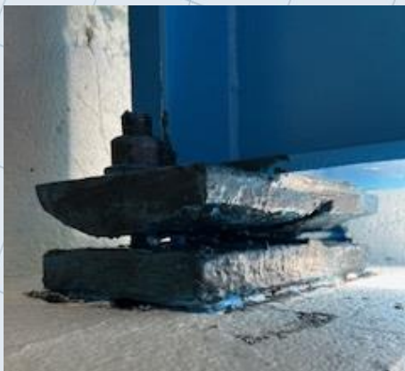
Bearing "floating" after corrosion removal
